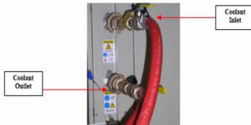
Figure 31 Coolant Water Interfaces
